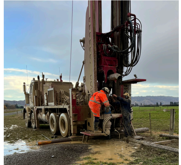
New monitoring bore installation by AIC
